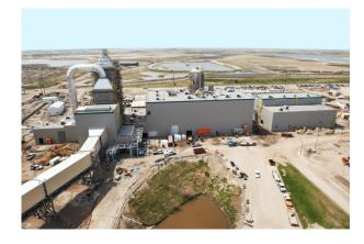
The same facility that strips carbon dioxide from the boiler's flue gas also captures sulfur dioxide (which it condenses into sulfuric acid to sell for industrial use) and scrubs out NOx. Fly ash from coal combustion is also captured and sold for industrial use. It's about as good as you can get for a coal plant, environmentally speaking.
