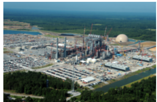
Kemper County plant under construction. Photo: Wikipedia Commons
