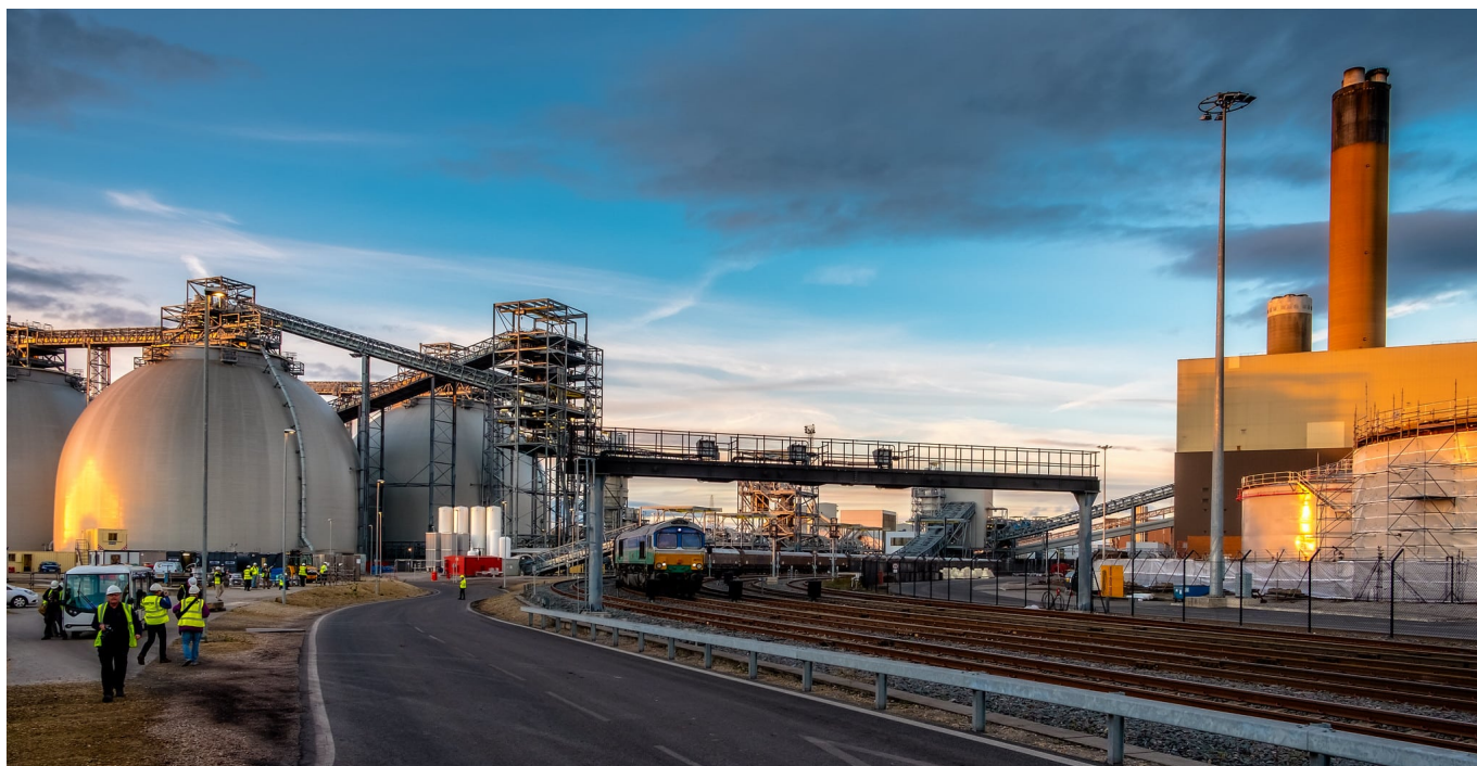
Wood pellet storage silos at Drax power station. Peter Leigh/Flickr
